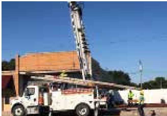
Prairie Land donated poles and sent crews to use the digger truck to set them. The poles are to support the panels for the new mural.
