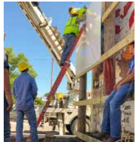
Students attached the supports for our crews to mount the heavy metal panels.
